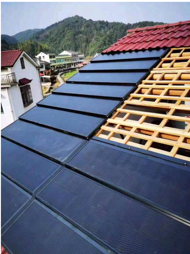
An example of an on-going installation of Flat solar tiles on a house roof.
