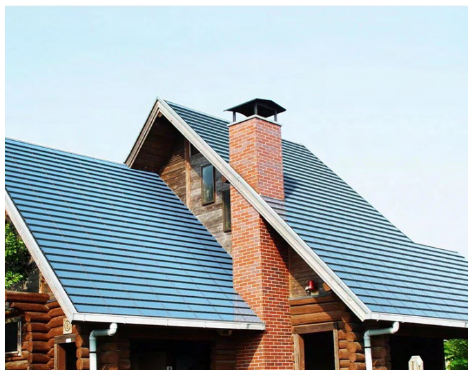
Completed installation of Flat tiles on house roofs.
